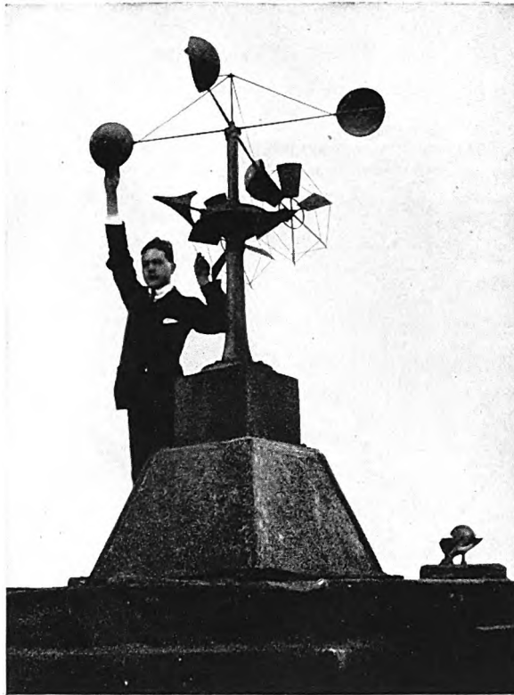
THE ROBINSON ANEMOMETER
