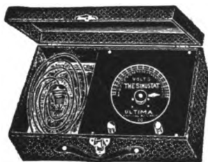
Fig. 247. Showing the No. 1 "Sinustat" Sinusoidal Current Controller, manufactured by Ultimo Physical Appliance Co. of Chicago.
