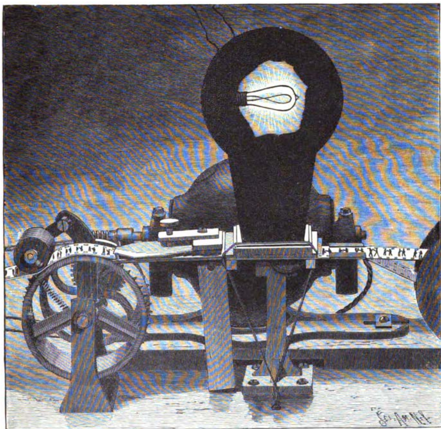
RIBBON PHOTOGRAPHY—EXPOSING AND PRINTING APPARATUS.
