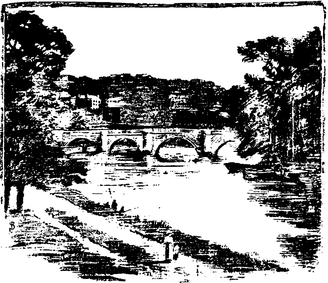
Richmond Old Bridge, from the foot of Asgill Road.
