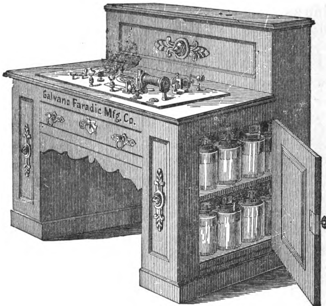
FIG. 11.—Cabinet Battery for Office or Hospital Use. (Galvano-Faradic Manufacturing Co.)
