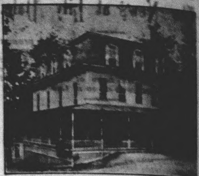
SOUTH PARK HOUSE.
