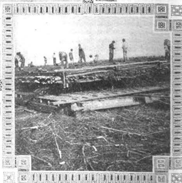
Building foundation mats for the new Southwest Pass jetties. Layers of willow brush are bound with scantling pinned together with hickory, no metal being used. They are built on sloping ways, launched, and towed into position, where they are sunk with stone into the mud of the bottom
