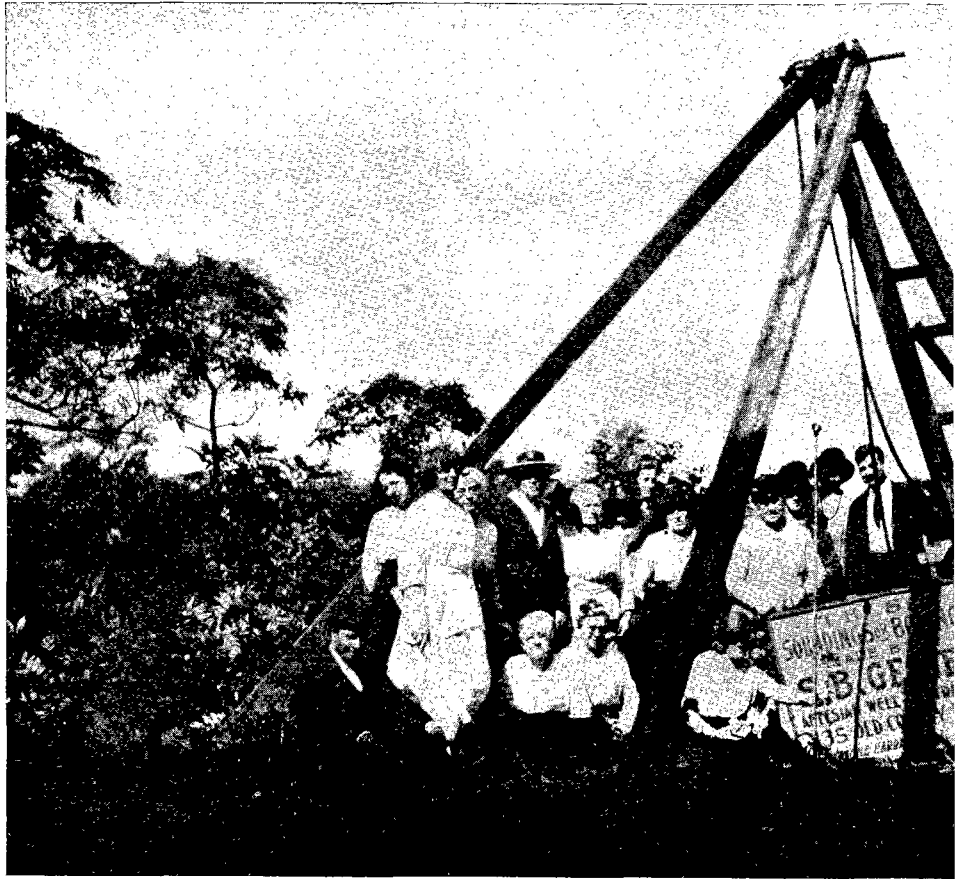
BAHAI FRIENDS AND WORKMEN ON MASHREKOL-AZKAR GROUNDS WHEN BORING C
