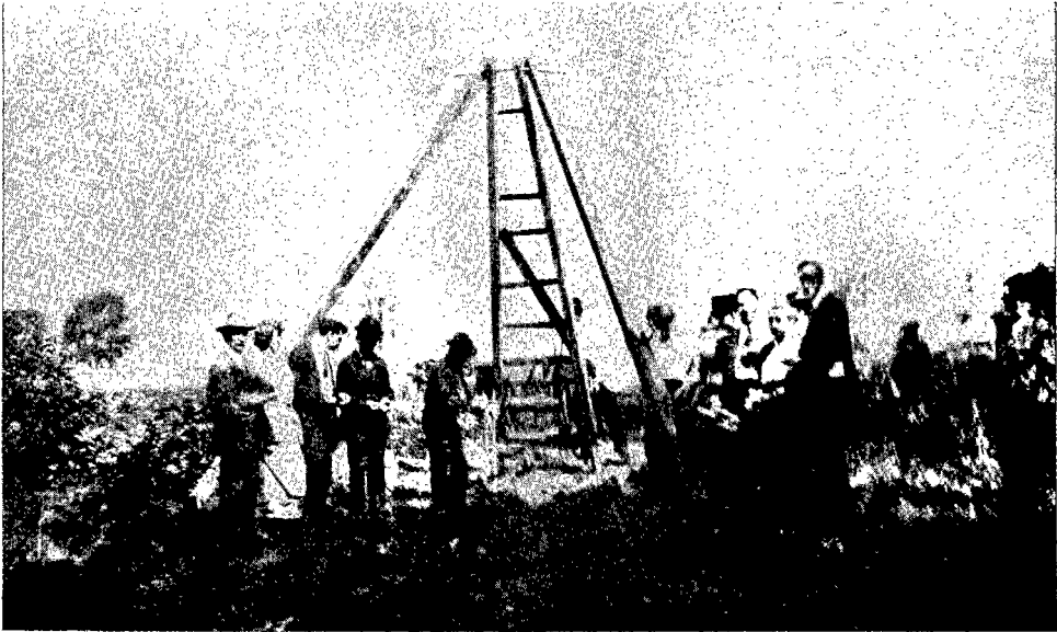
BEGINNING FIRST BORING—FRIENDS HOLDING SOIL IN HANDS
