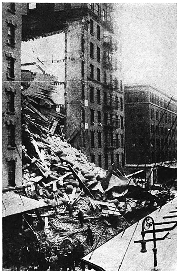
The lives of many workers were endangered when an over-loaded floor precipitated about two million dollars' worth of merchandise to the street below. Such accidents are decreasing with the more extensive use of safeguards.
