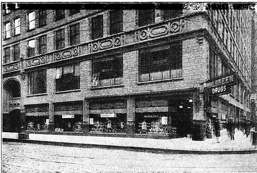
The Walgreen Store at 199 Franklin Street, Chicago.
