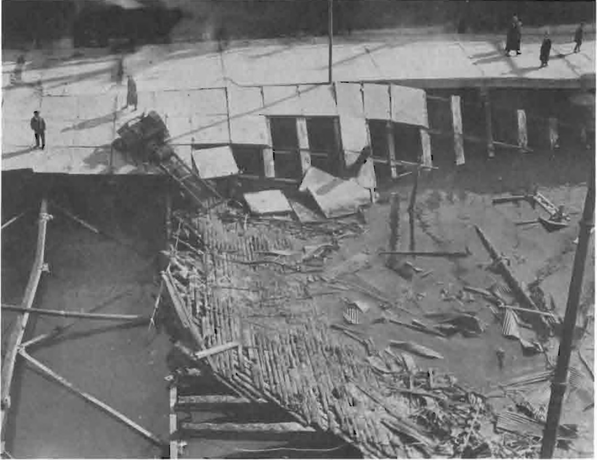
One of the docks that collapsed in Yokohama as a result of the earthquake. Photograph by Manly P. Hall.
