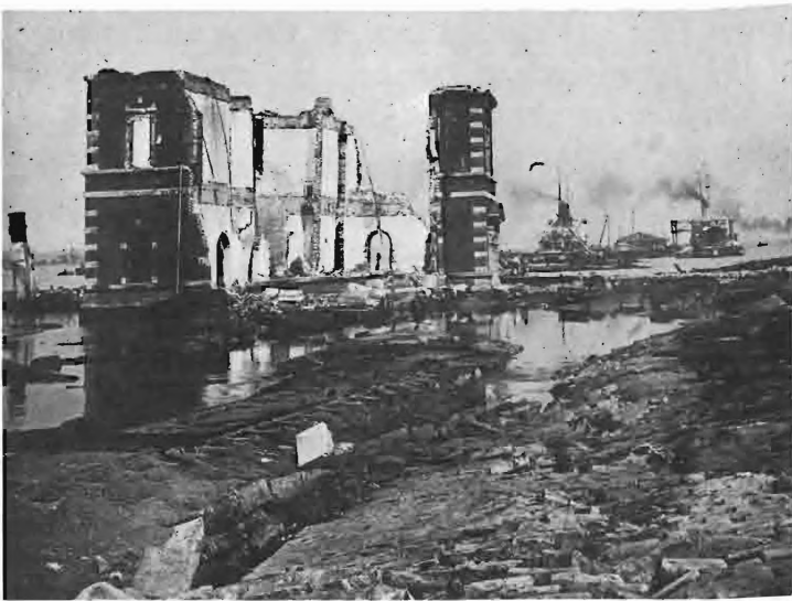
Scene in the Port of Yokohama a few weeks after the great earthquake of 1923.
