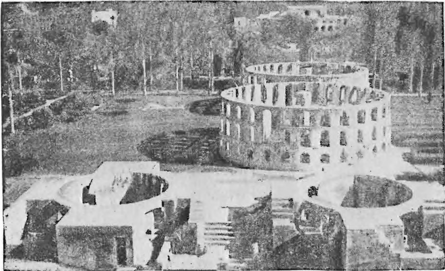
The Ram Yantra, two circular buildings forming one instrument for the measurement of altitude and azimuth. From a handbook of the astronomical observatory at Delhi by Lala Bholanath, B.A., L.C.E.
