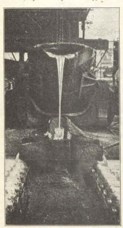
View of Ladle Emptying Molten Metal into Moulds, Pig Iron Machine, Pittsburg
