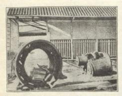
Westinghouse Engine Exposed to Weather on Account of Destruction of Packing—Box Destroyed and Many Studs on Cylinders Broken
