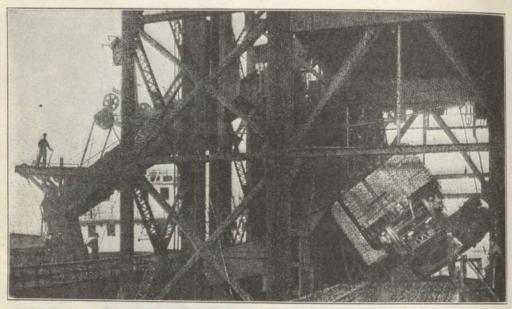
Dumping Whole Cars of Coal into Hopper to Be Poured into Vessel's Hold at the Rate of About 25 Cars Per Hour, Conneaut, Ohio
