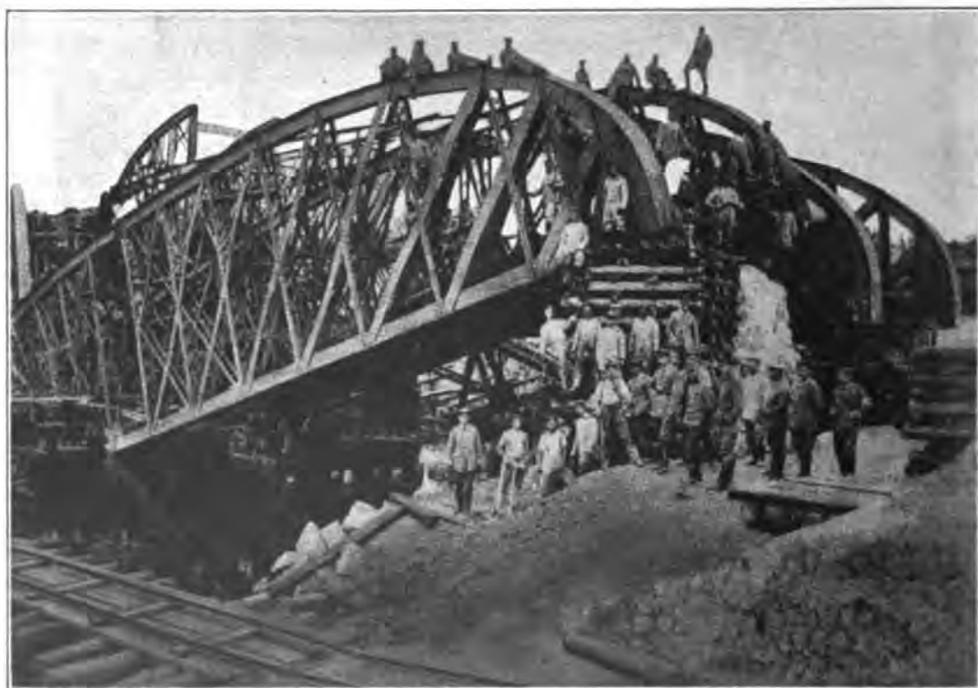
GERMAN PIONEERS RECONSTRUCTING A BRIDGE IN GALICIA.
