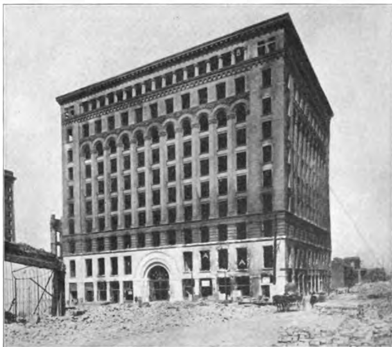
A BRICK BUILDING WHICH HAS WITHSTOOD INTENSE HEAT, 500° The brick and terra cotta walls are virtually unscathed.
