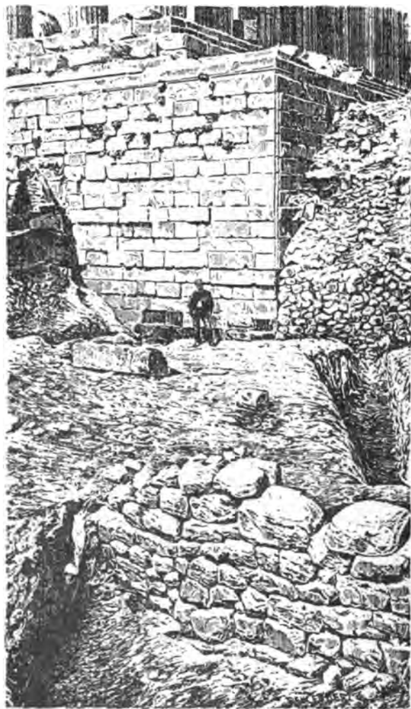
THE ARTIFICIAL FOUNDATION OF THE PARTHENON LAID BARE. FURTHER DOWN THE PELASGIAN WALL.
