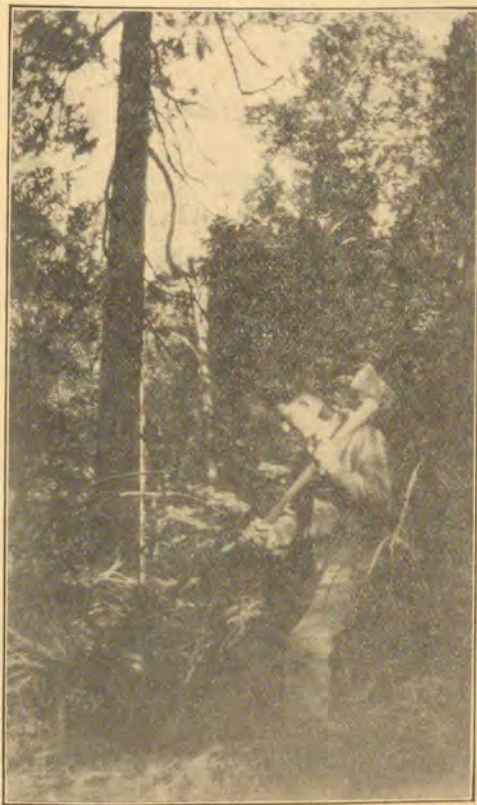
Clearing Ground for Cabin Site
