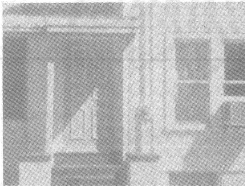
Side view of N.S.A.C. Headquarters.
