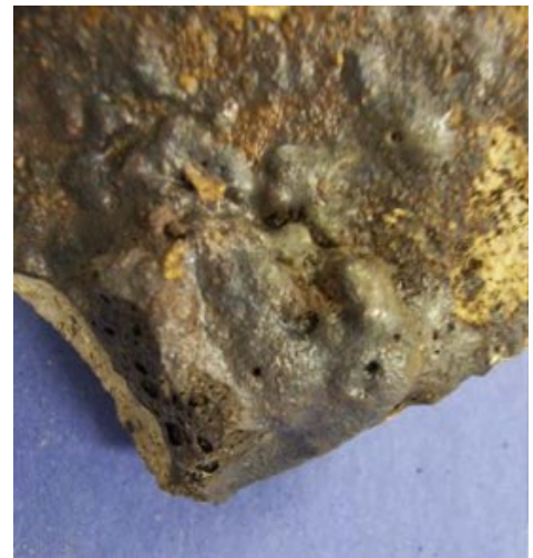
Brick—Burned area, closeup
