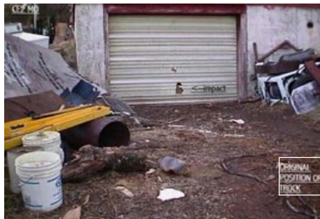
The driveway and garage door that truck was pushed into. Notice hole.
