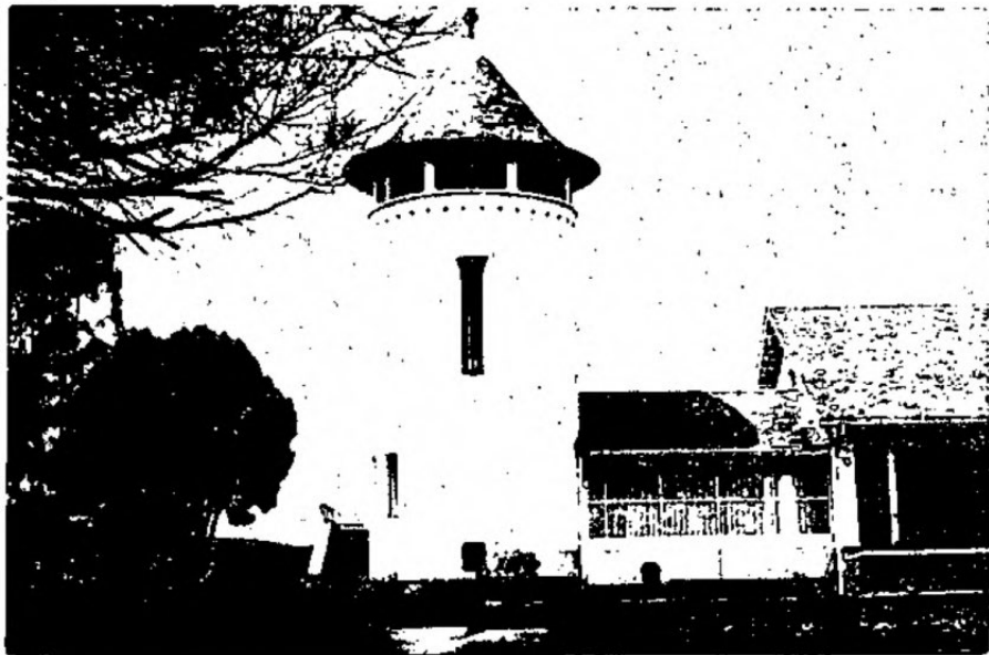
Observation Tower at La Rochelle
