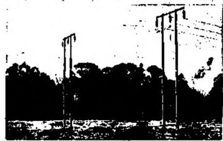
Electric power lines within few meters of landing site.
