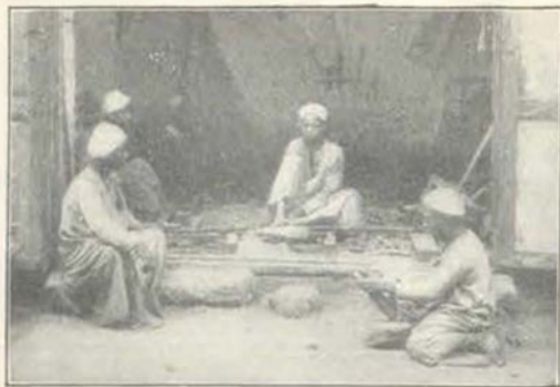
NATIVE CARPENTER SHOP.
