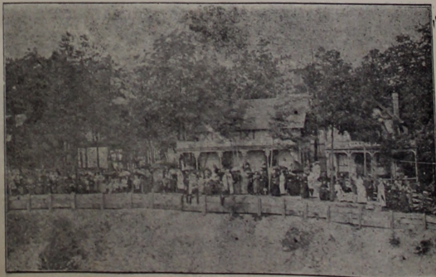
LAKE PLEASANT—HEADQUARTERS BUILDING.
