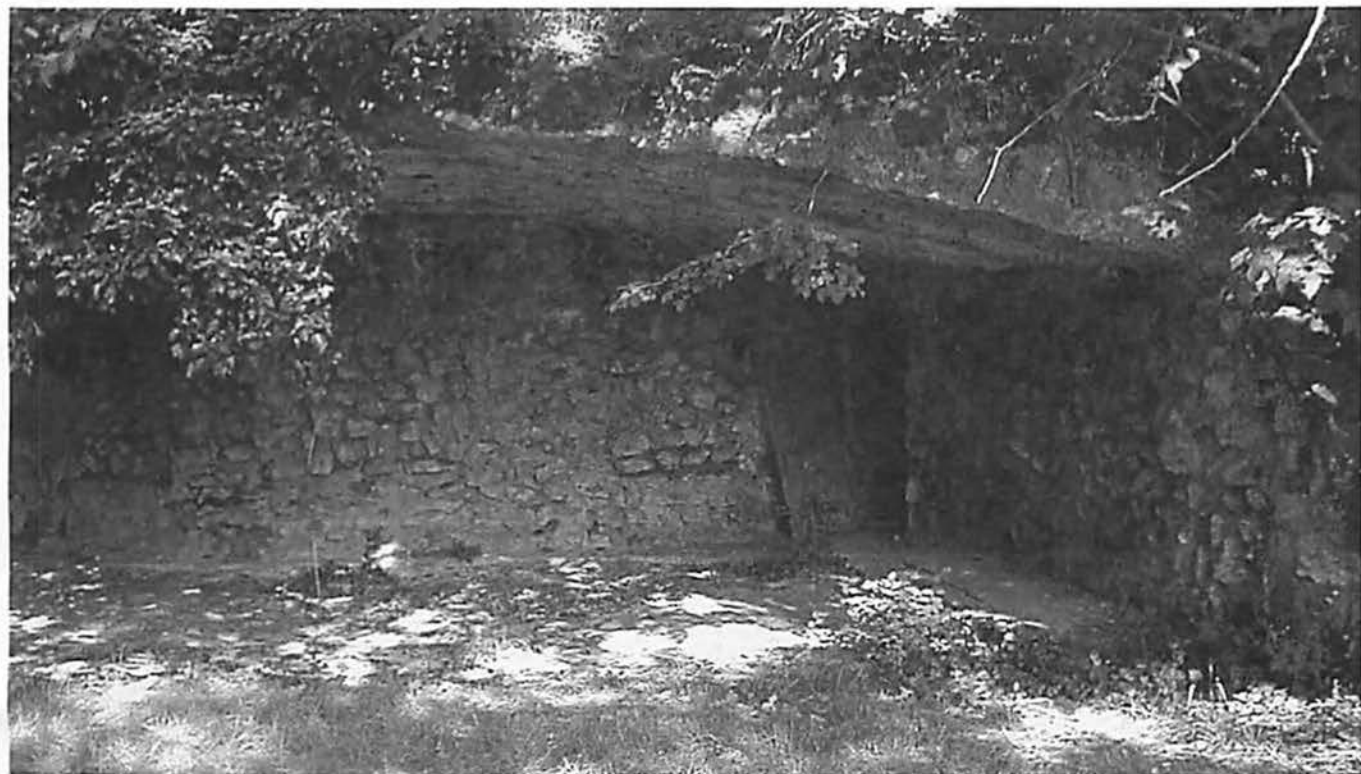
The bath-house at the Prieuré was built into the side of a small rise, sunk into the earth.
