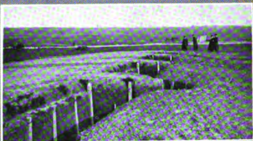
Note How the Trenches Zig-Zag For Additional Protection
