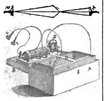
The instrument is fitted into a neat Mahogany case (with lock and key) 8 inches long, 4 wide, and 3 deep.
