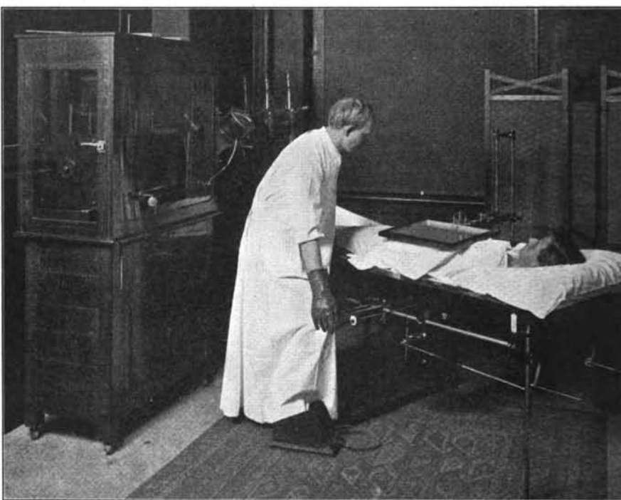
Employment of the Klinoscope for stomach and bowel observations, patient lying. Twelve-inch coil to the left, X-ray tube beneath the patient, and easily operated by the observer's right hand.
